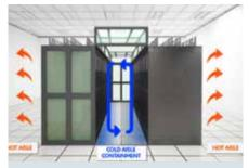
Standard co-location cabinets with cold aisle containment technology
